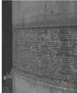
Figure 3 – Close-up of texture resulting from a single 8 inch wheel path grind.
