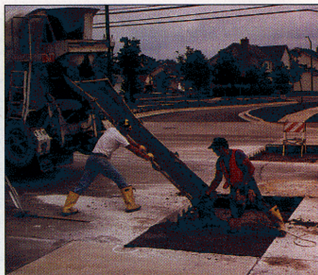
Full-slab replacement is one procedure of the CPR maintenance system
