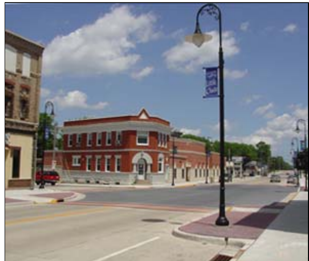
Main Street in the Village of Little Chute, Wis., is a collector street. It features traditional concrete pavement, colored and stamped concrete pavements; and colored and imprinted sidewalks. The recent reconstruction project was recognized by ACPA with an "Excellence in Concrete Pavement" award.
