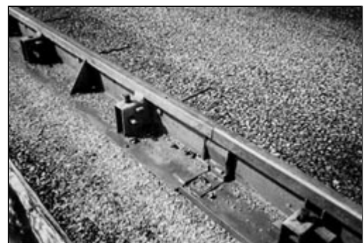
Forms should rest on a level surface and be securely pinned in place.
