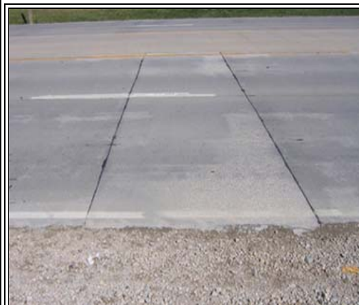
Figure 3 - A full-depth patch in a highway is typically placed at deteriorated transverse joints or cracks, and is usually at least one lane wide.
