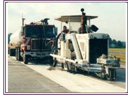
Diamond grinding improves surface characteristics and environmental benefits of concrete pavements.
