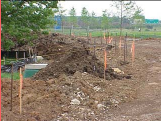
The set up and maintenance of the stringline, including stringline material, stakes, staking interval, splices, and repositioning frequency all may impact the resulting pavement surface.
