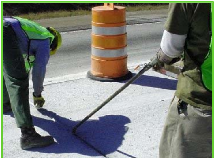
A few simple steps will assist with proper placement or replacement of joint sealants.
