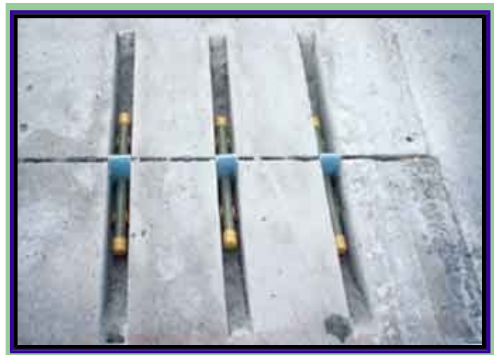
Dowel bars are a design element that impact long-term pavement performance and can be retrofit into undoweled pavements.
